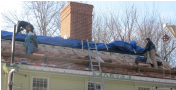
Talented craftsmen brave the cold temperatures to install the Certi-label™ roof
