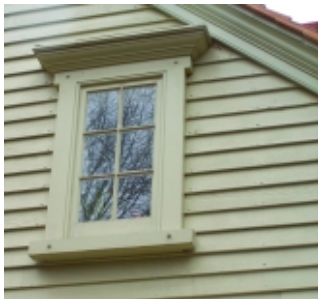
Window molding detail
